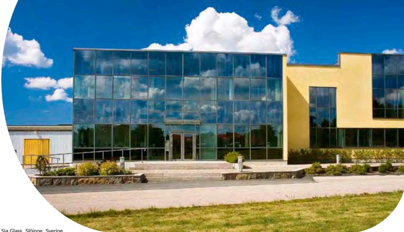
Sia Glass, Slöinge, Sverige. Pilkington Spandrel Glass Coated Pilkington Suncool™ 50/25
